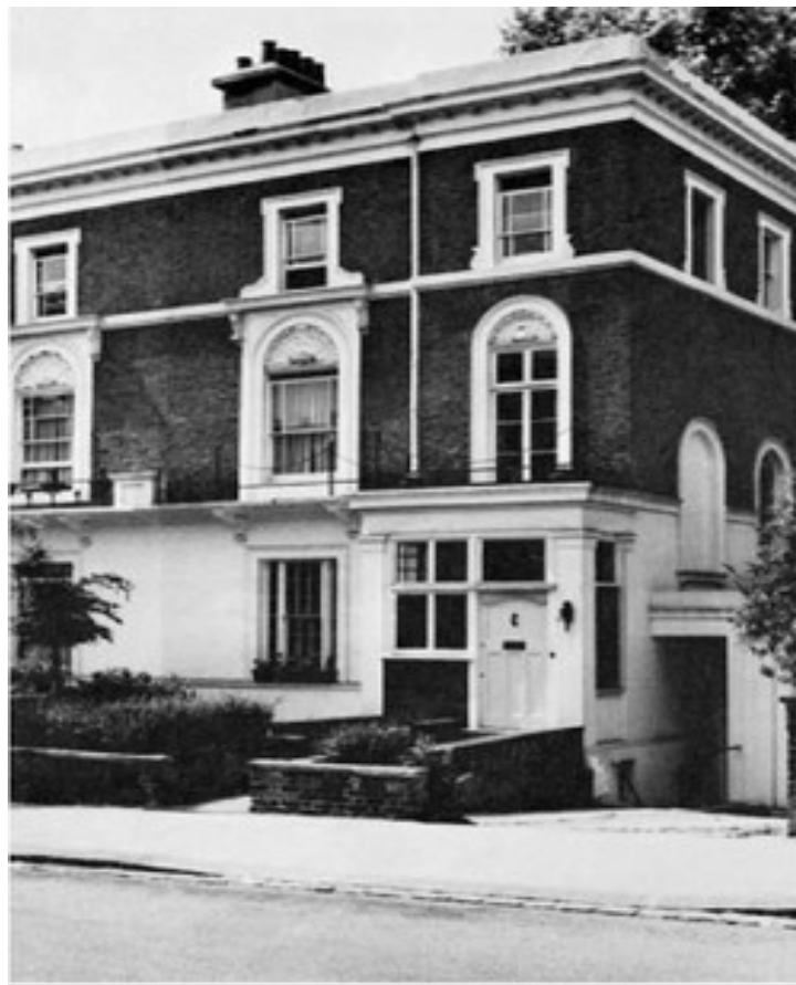
17 Lansdowne Road, Fassade, 1957
